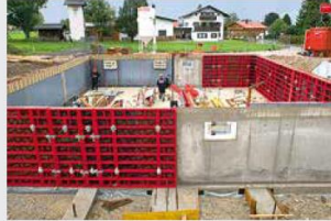
Wall Formwork
